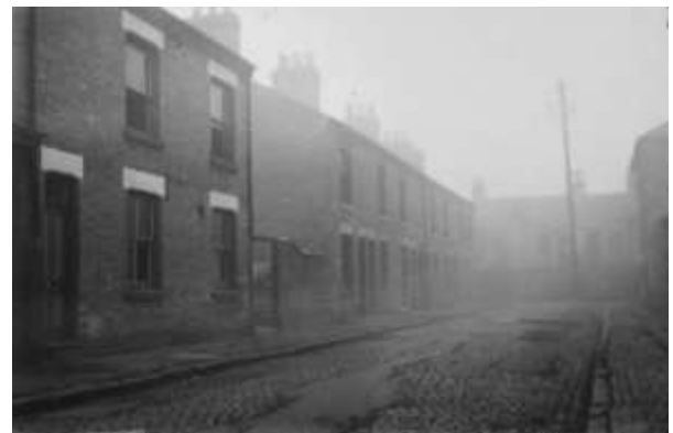
Liggins Street before demolition
